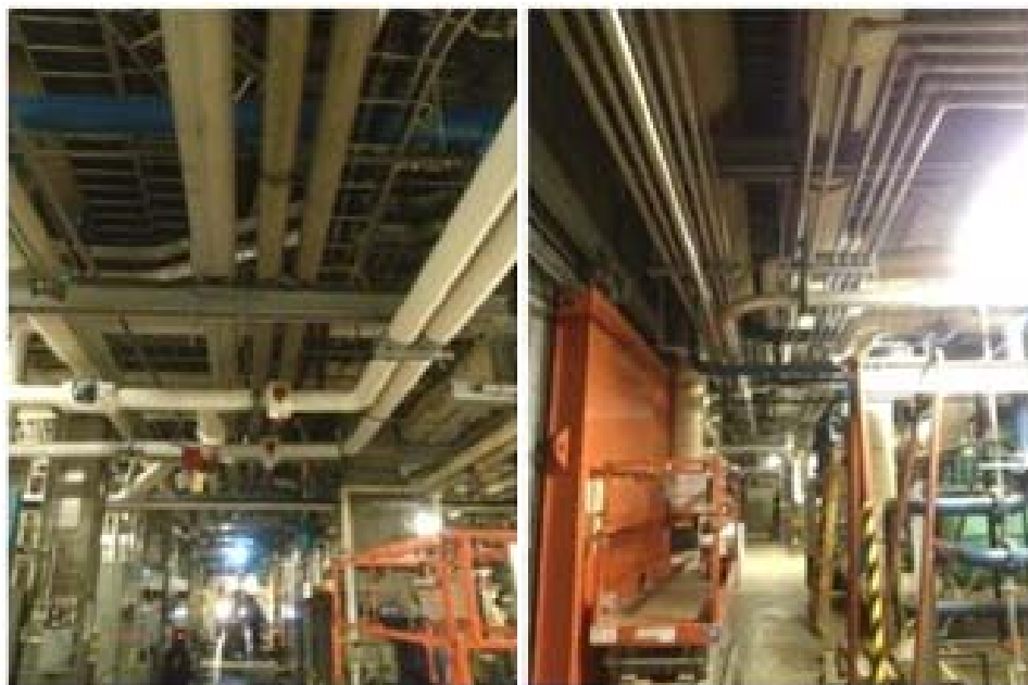
NBI Deionized Water Piping Installed
