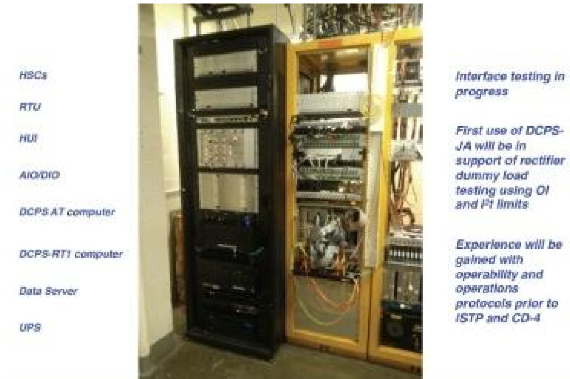
Junction area DCPS complete
