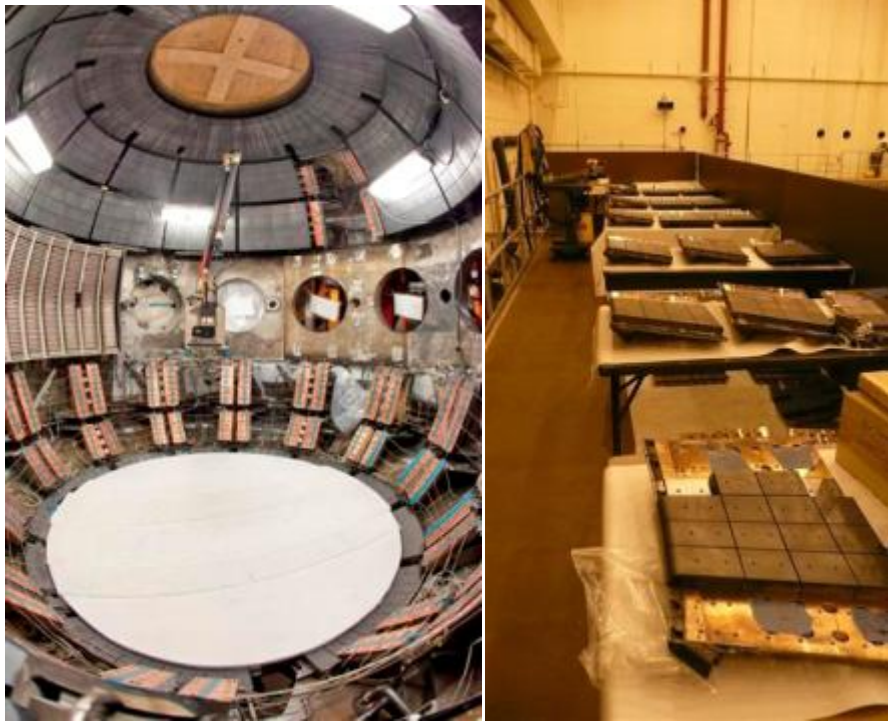
Lower Passive plates being installed
