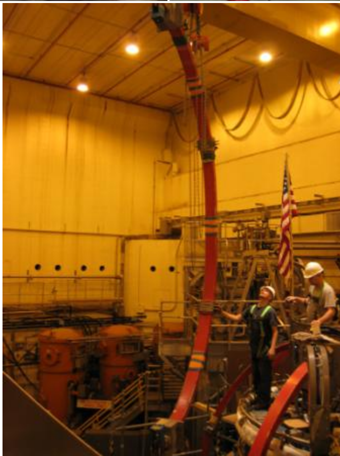
Two new outer TF coils fabricated and installed
