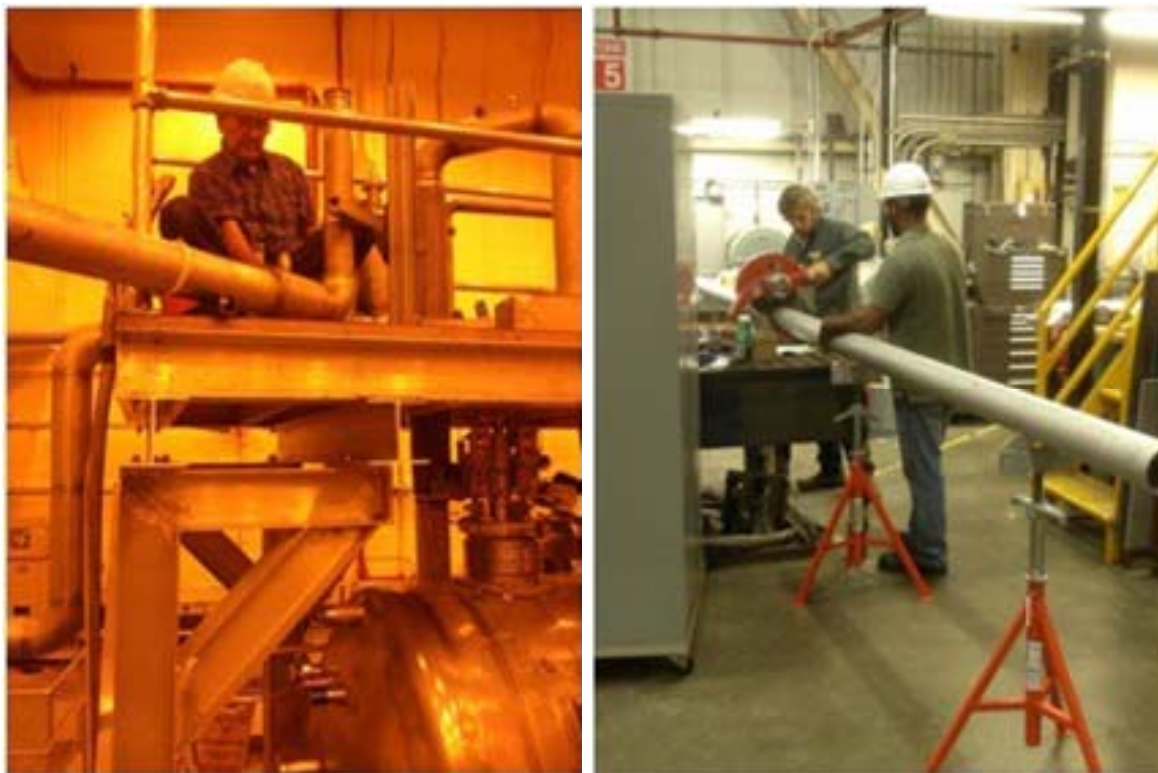
Cryogenic LN and LHe Piping installed
