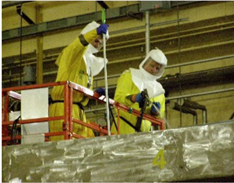
Box decon from lift and from source platform using 25 gallon sprayer and DI water
