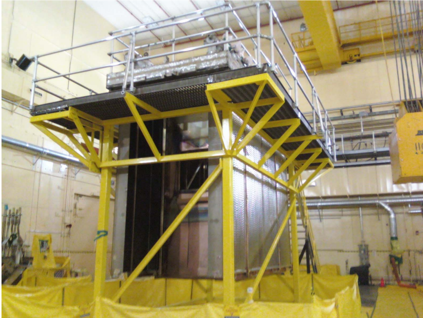
Lid and cryo panels sitting in new stand... ready for decontamination phase
