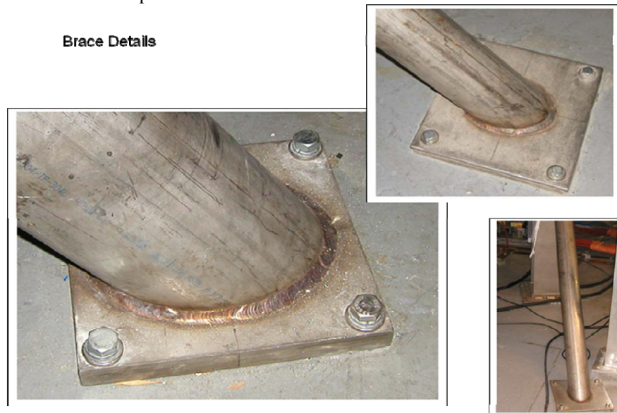
Figure 12.15.1-2 Brace Pad Details
