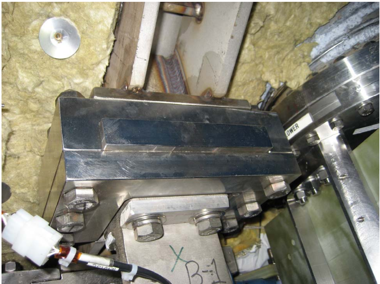
Figure 9.8-2 Welds at Umbrella Foot Plate
