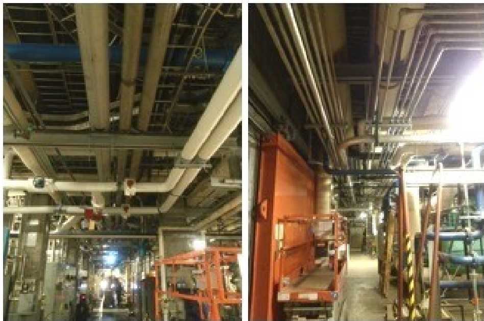
NBI Deionized Water Piping Installed
