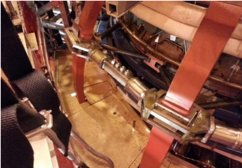
Outer TF Leg turnbuckle supports
