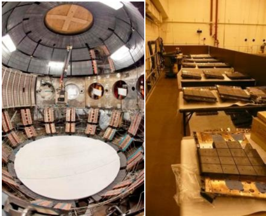
Lower Passive plates being installed
