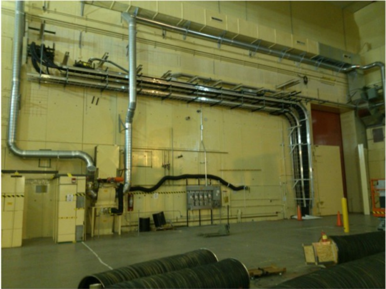
Power Cables in TCB,TTC to NTC Installed
