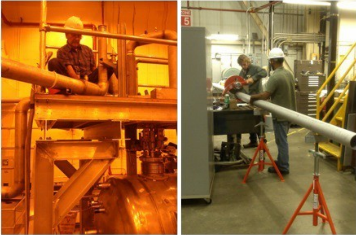
Cryogenic LN and LHe Piping installed
