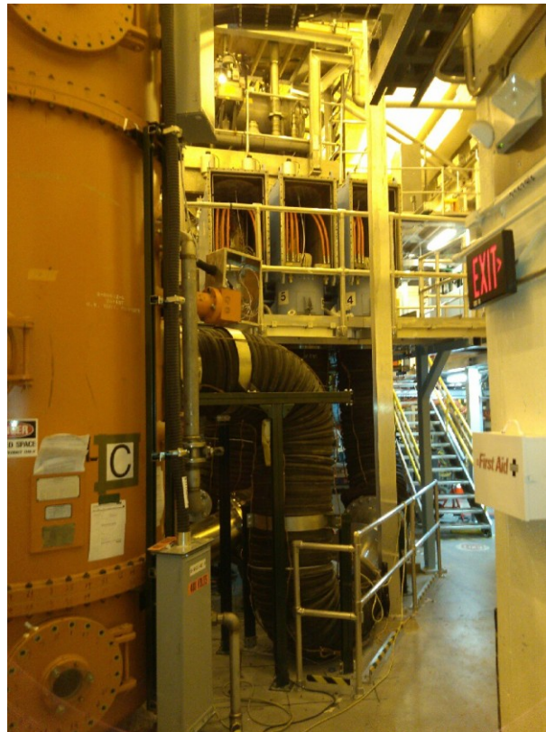
Transmission Lines Installed
