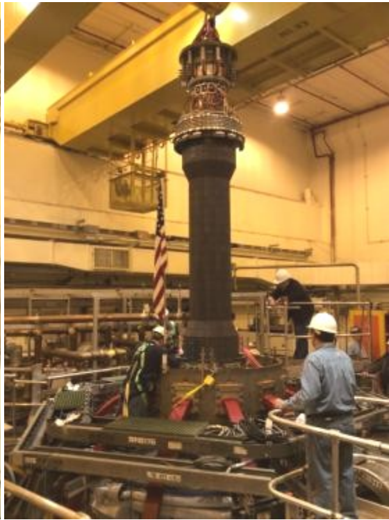
CS assembly being lifted into the machine
