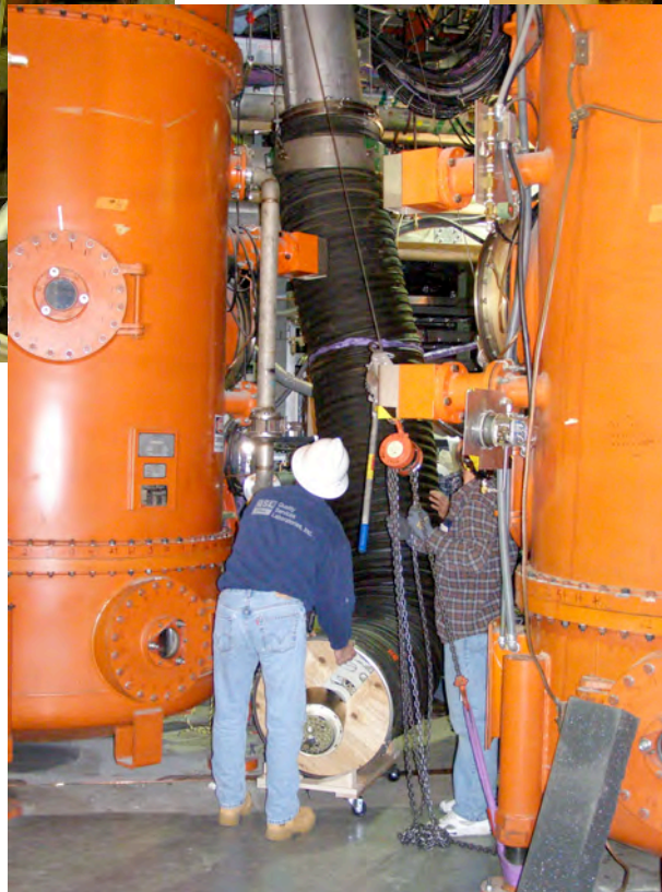
Saving N4 Xmsn line for reuse
