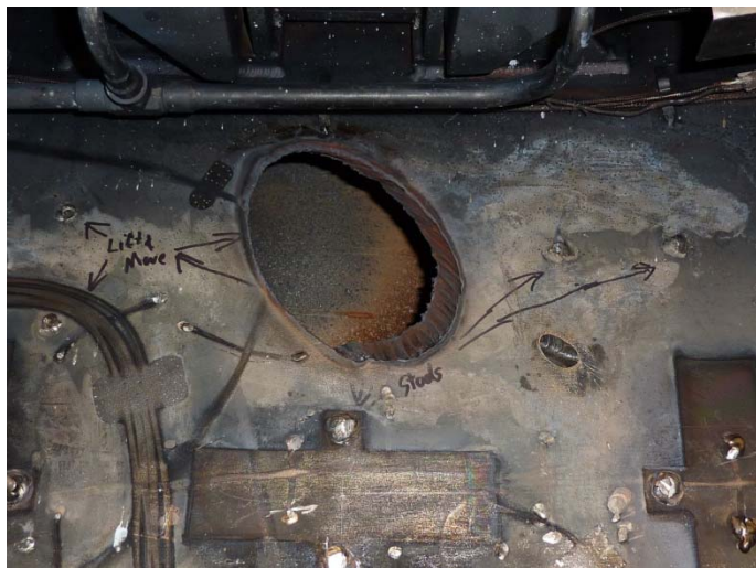
Wire brushing of cut
