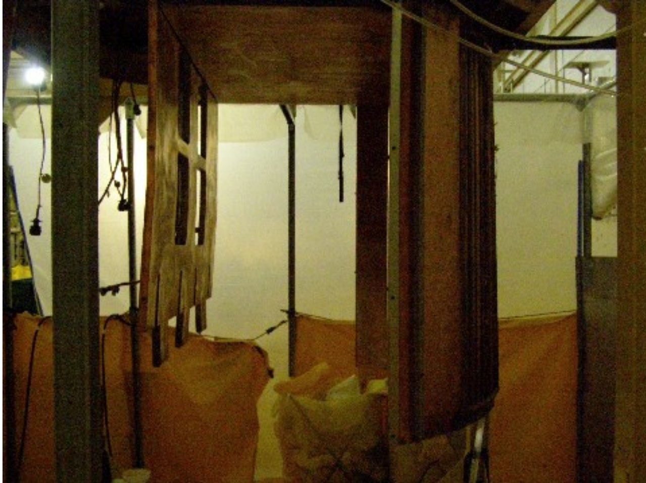
Ion Dump - louvers removed for decon in fume hoods
