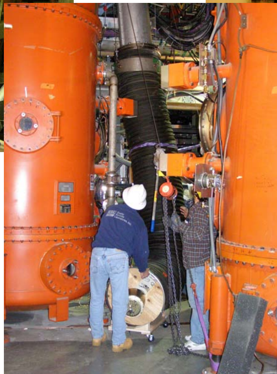
Saving N4 Xmsn line for reuse
