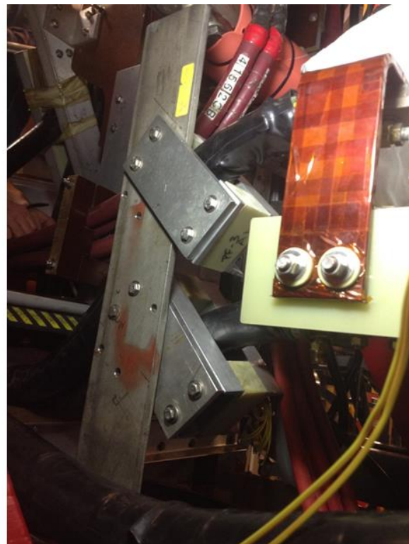
Figure 4.0-12 Representative Flex Cable Restraints [14]
