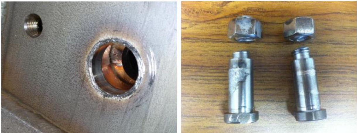
Figure 3.10-1 Photo showing the arcing on bolts and stainless steel plates
