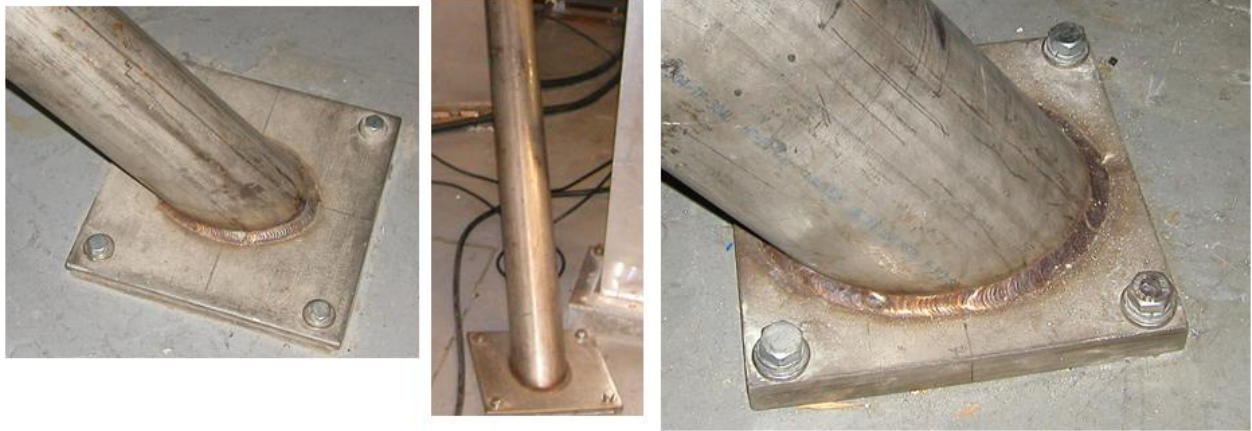
Figure 8.2-2 Brace Welds and Hilt' Cap Screws.
