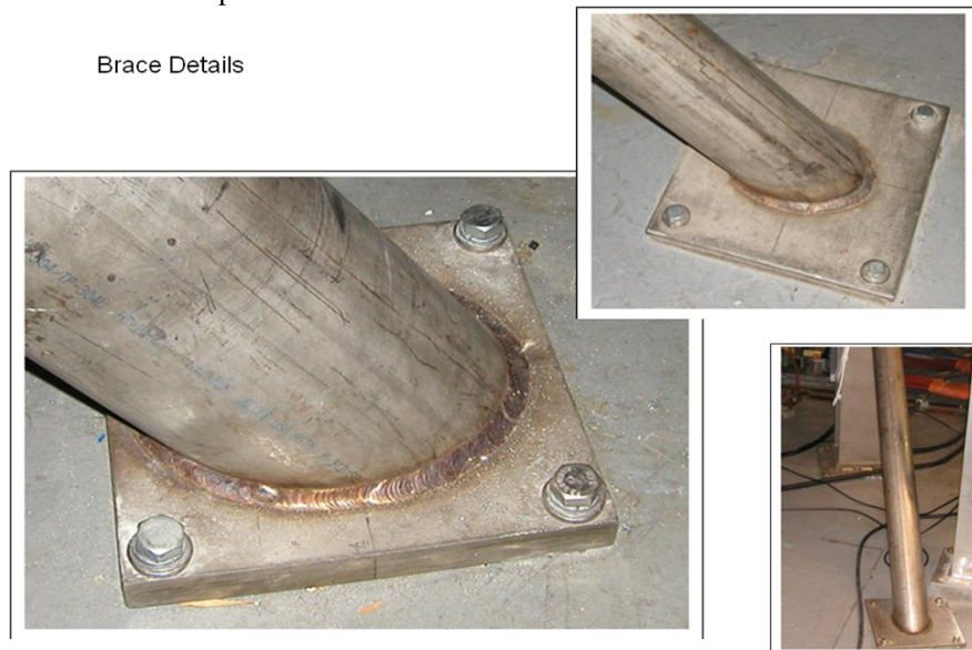
Figure 12.15.1-2 Brace Pad Details
