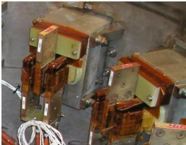
Figure 7.1-2 View Inside Umbrella Structure
