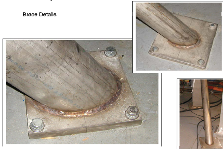
Figure 12.15.1-2 Brace Pad Details
