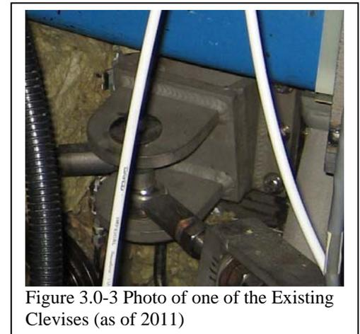
Figure 3.0-3 Photo of one of the Existing Clevises (as of 2011)
