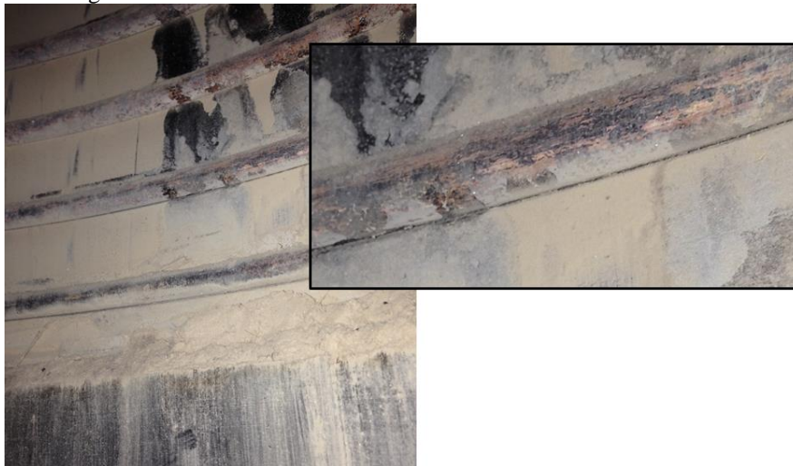
Figure 4.4-5 Centerstack Casing Cooling Tube Disruption Photos Taken Dec 14 2016
