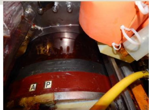
Figure 4.0-3 Lower OH Ground Paint Connection
