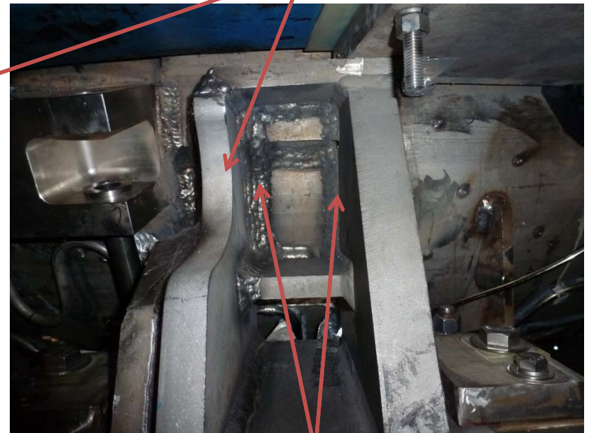
Welded inside contact areas
