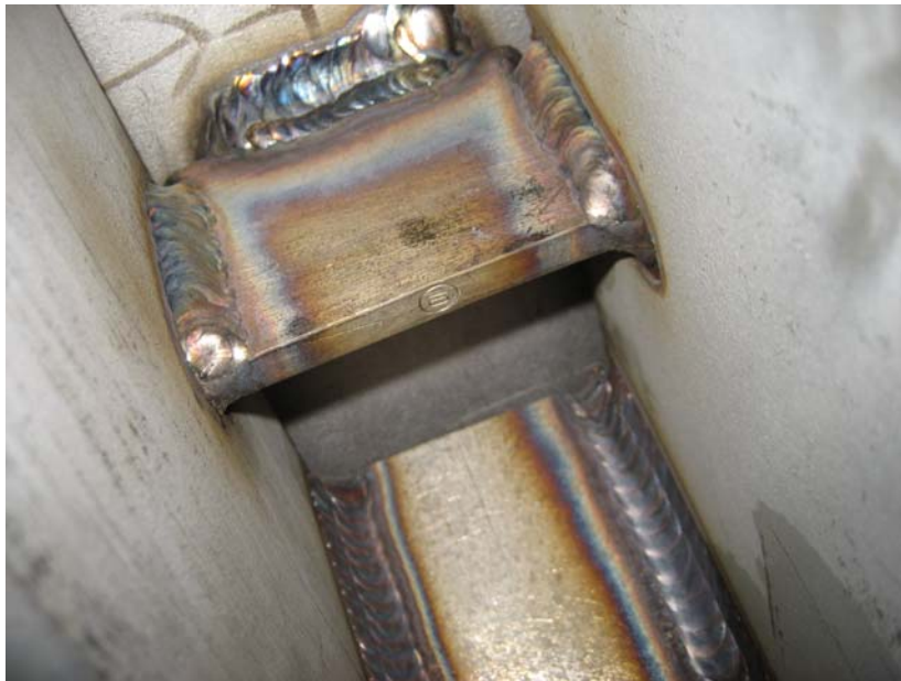
Figure 5.5-2 Photo of the One of the Tabs that Connect Rib Pairs
