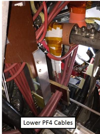
Figure 10.1-1 As-Builts of the PF4 Terminals and Cables
