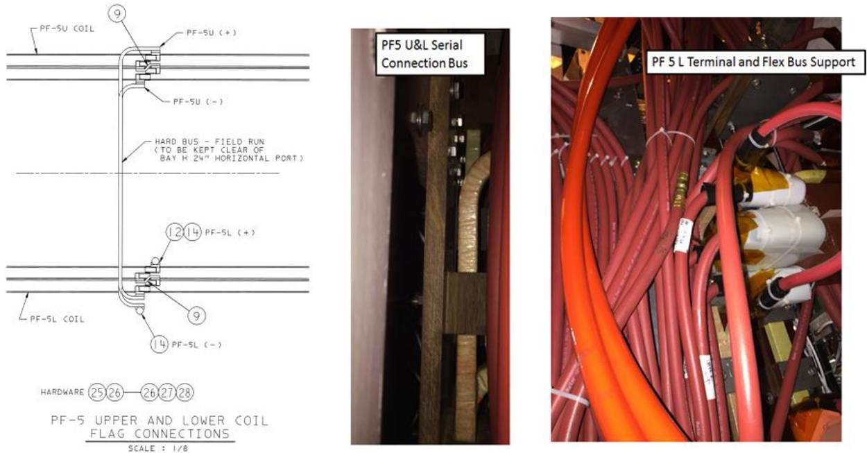
Figure 10.1-3 Series Connection Bus Between Upper and Lower PF5
